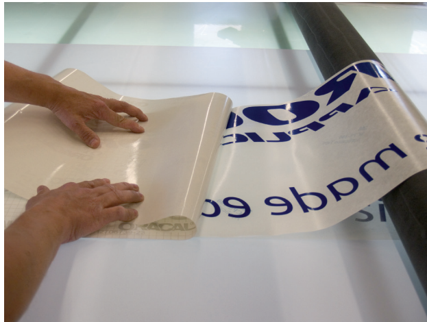
11. Apply the other half of the graphic using the pressurised roller.
